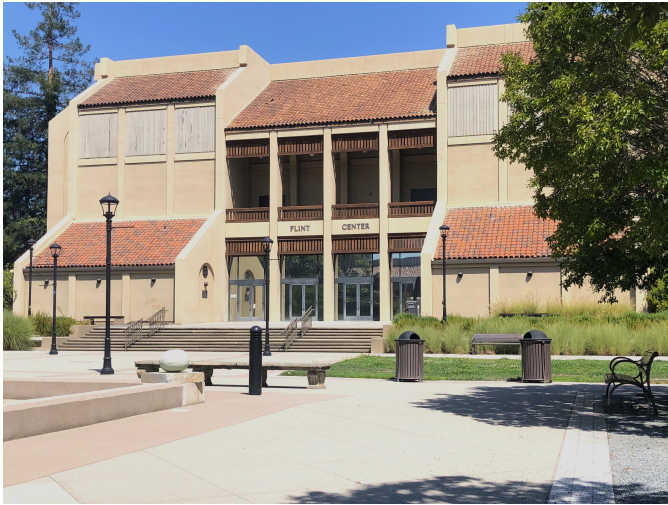
A. Flint Center south elevation (entrance)
