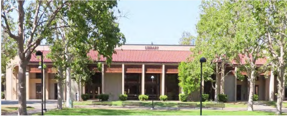
Photograph 32. View of Map ID 32. S8 east (main) elevation, facing northwest.
