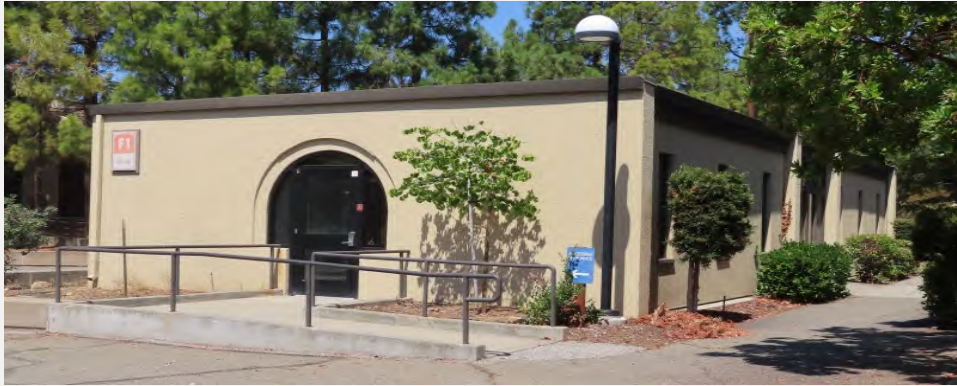
Photograph 11. View of Map ID 16. F2's south and east (main) elevations, facing northwest.
