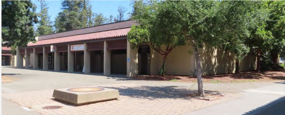
Photograph 23. View of Map ID 23. L7 west (main) elevation, facing southeast.
