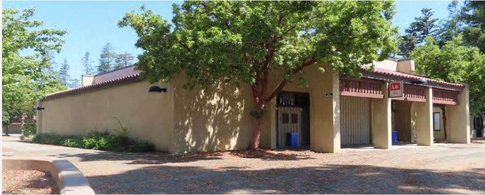
Photograph 20. View of Map ID 25. L8's south (main) elevation, facing northwest.
