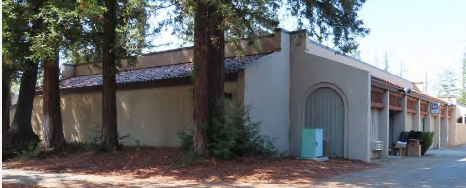
Photograph 35. View of Map ID 37. S5 east (main) elevation, facing northwest.
