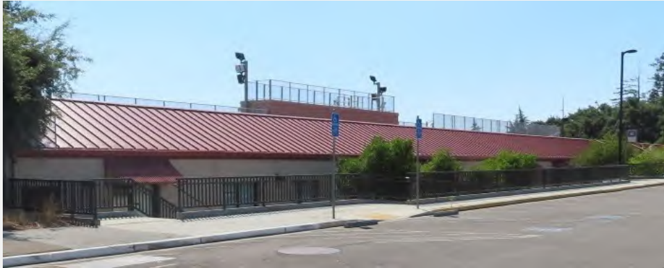
Photograph 47. View of Map ID 53. Stadium and Track G, facing northeast.
