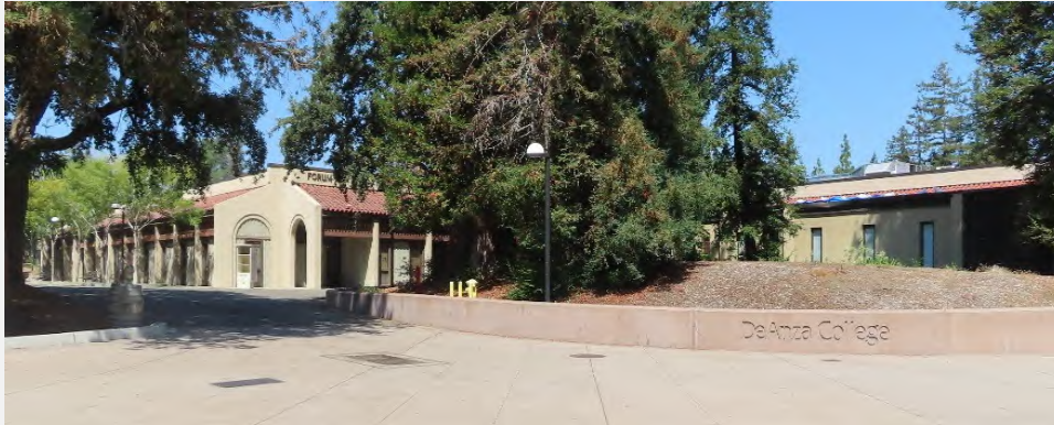
Photograph 2. Map ID 5. A1, showing the buildings' main (south) and west elevations, facing northeast.
