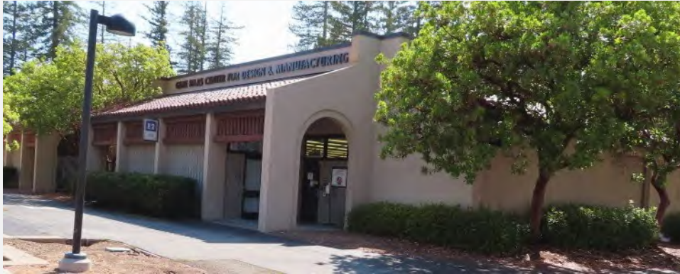
Photograph 38. View of Map ID 38. S3 west (main) elevation, facing southwest.
