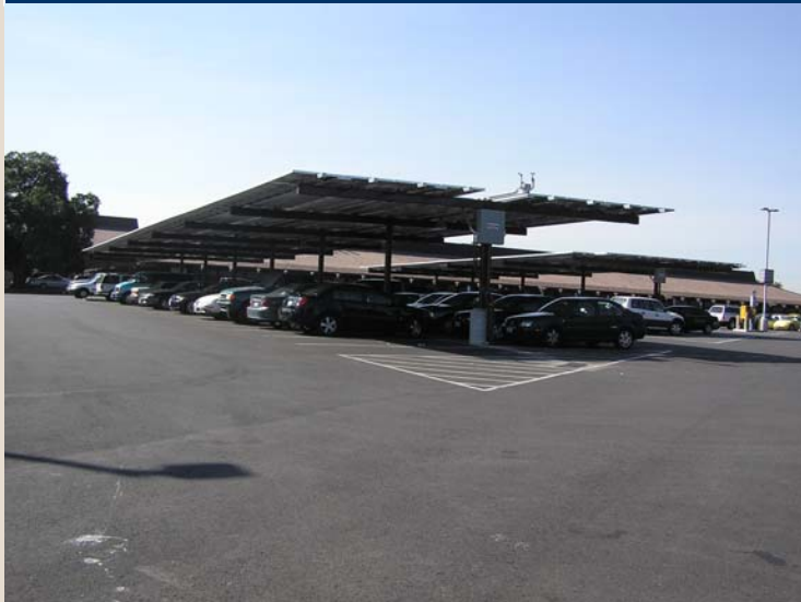
PV Shade Structure
